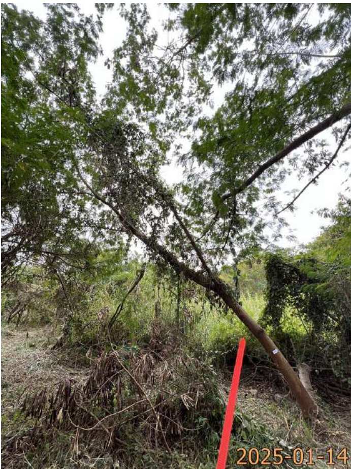
T22 (Overview) (Leaning)
