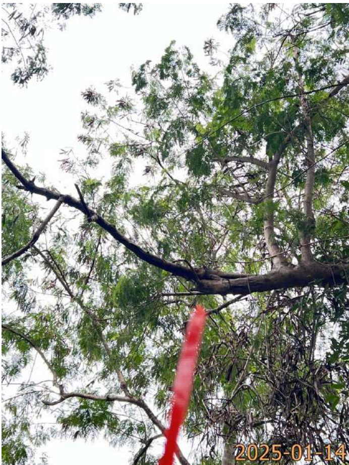
T8 Broken trunk
