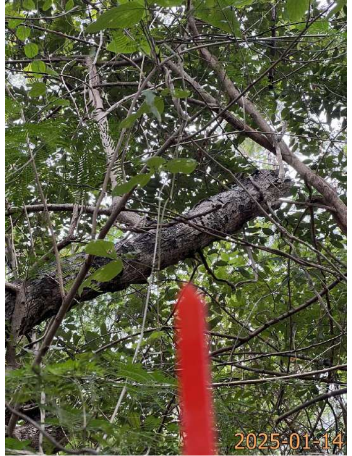
T1 Broken trunk
